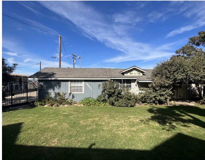
Overview of South Elevation
