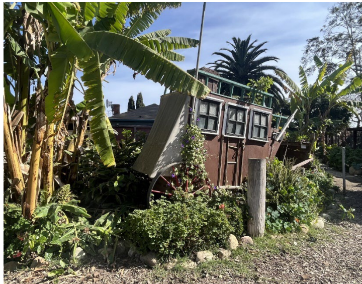
Representative Photograph-Contemporary Interpretive Structures
