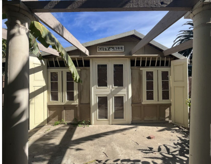
Representative Photograph-Contemporary Interpretive Structures
