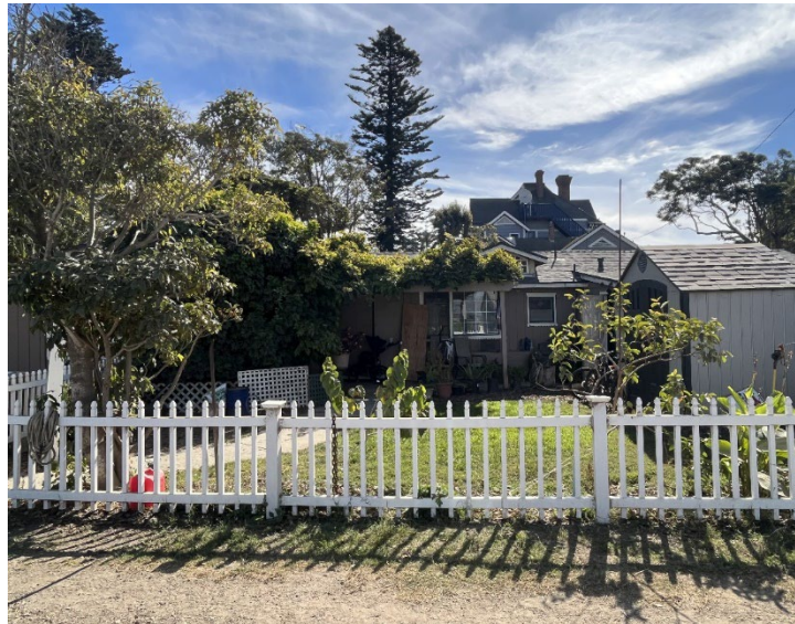
Overview of North Elevation
